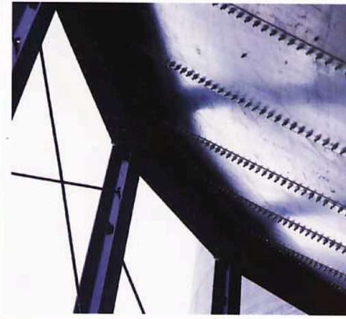
The bin is connected to the hopper cone via a rugged compression ring that ties the entire structure together securely. Note as well, the heavy-duty tie rod braces for added integrity and reliability. (ABOVE)
